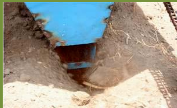
Subsoil coir pith applicator in operation
